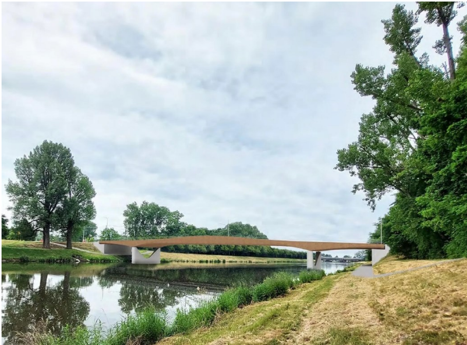
Fig. 6. New look of Kapitán Bartoš bridge [12]
