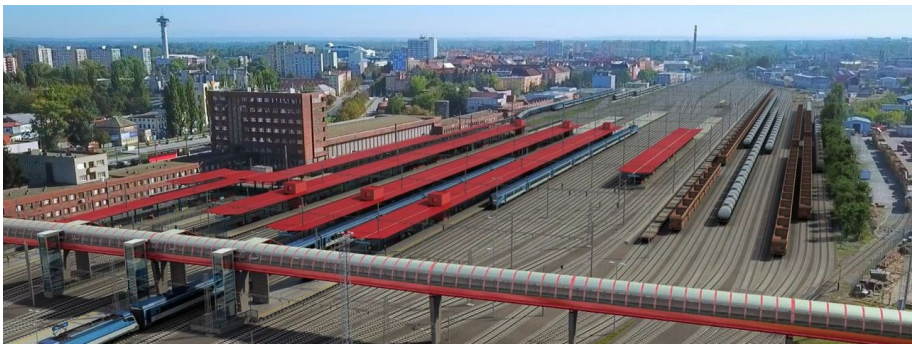
Fig. 3. Pardubice junction after the reconstruction [4]
