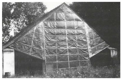
**Figure 8.** A wall collector for drying agricultural products Source: (Niemiec, Król, 1994b, p. 1).
