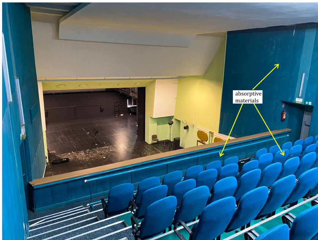
Figure 7. View of the interior of the hall from the balcony; sound absorptive finishes are marked with yellow arrows.
