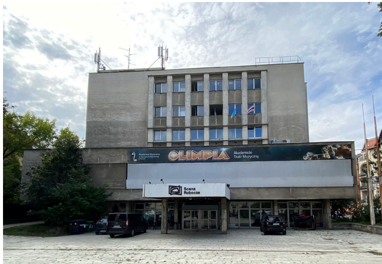
Figure 1. View of the building.
