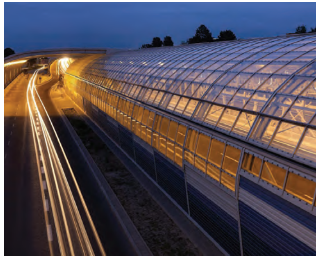
Fig. 7. External view of the half-tunnel noise barriers [14]
