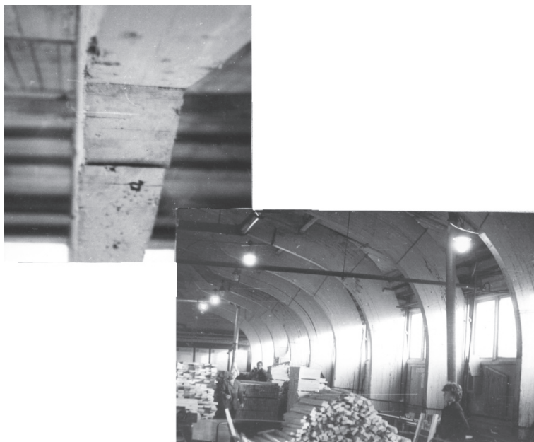
Fig. 2. The nature of the defects of GLBFs with a ledge in the crossbar during operation
