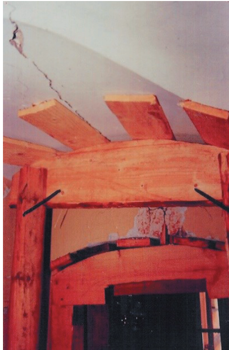
Fig. 4. Fragment of supported roof in the cloister
