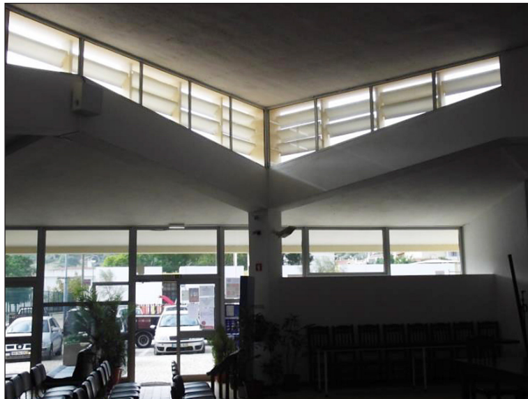
Figure 4. Aspect of the interior of the building.
