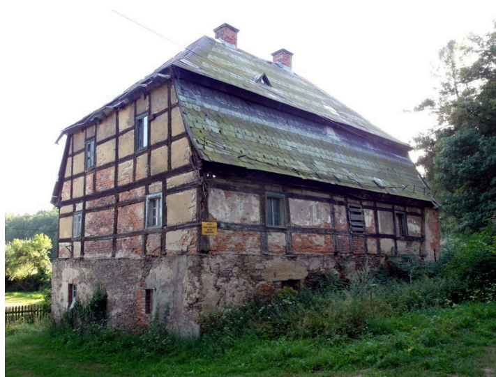
Figure 2: A mansard roof, four-slope with lower-half-gable, a false rafters on both levels of the slopes and a tiny dormer topped with two-slope roof, Owiesno, Lower Silesian Voivodship (2013), photo by the author
