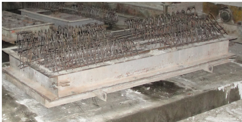
Fig. 1. The general view of reinforcement ( own research )
