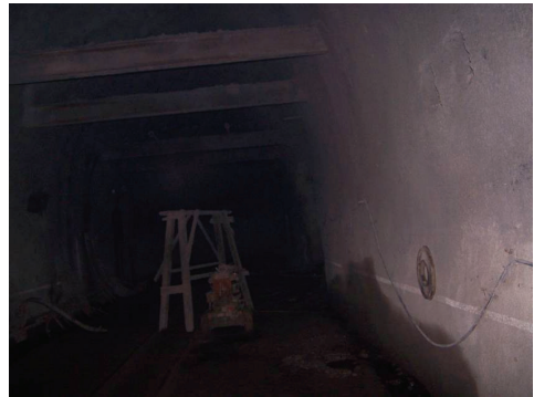
(b) Pump house
