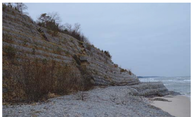
Fig.4. Degradation of reinforced cliff part at Jastrzebia Gora – situation of January 2017.
