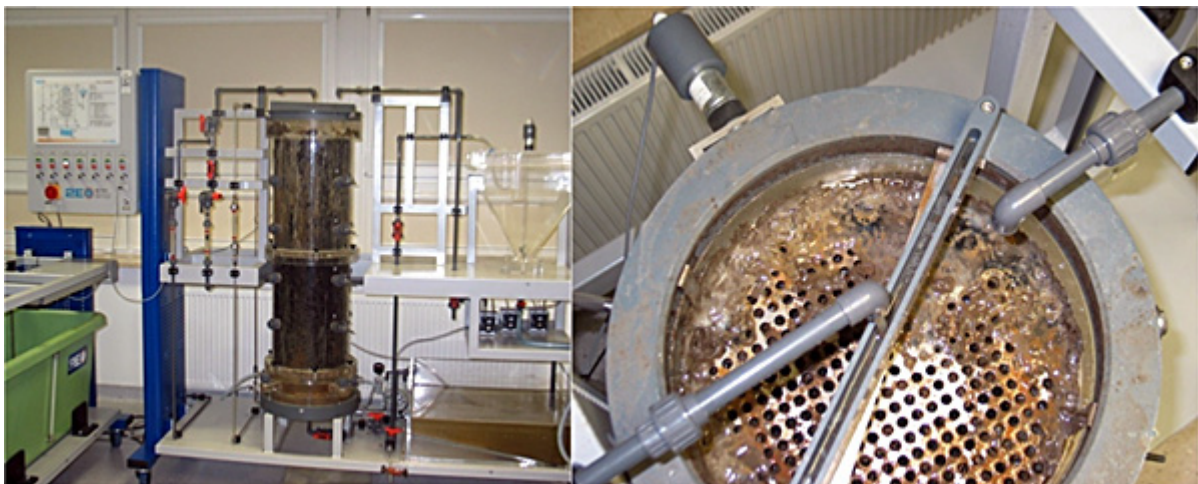
Figure 3. Research installation with main elements during operation (Nov 2017)
