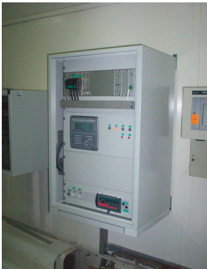
Fig. 2. The microprocessor electro-hydraulic power controller (MREH) made by "ITC"
