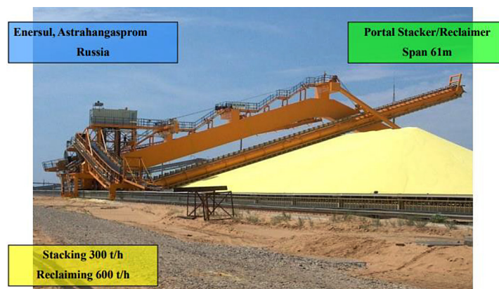
Fig. 6. The Enersul stacker (capacity 600 t/h)
