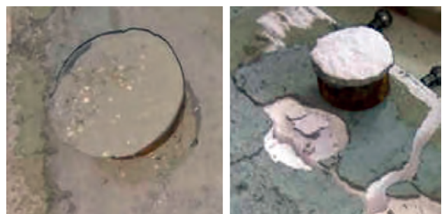
Fig. 10. Damage during adhesion tests on non-incised samples of concrete (left) and aerated concrete (right)
