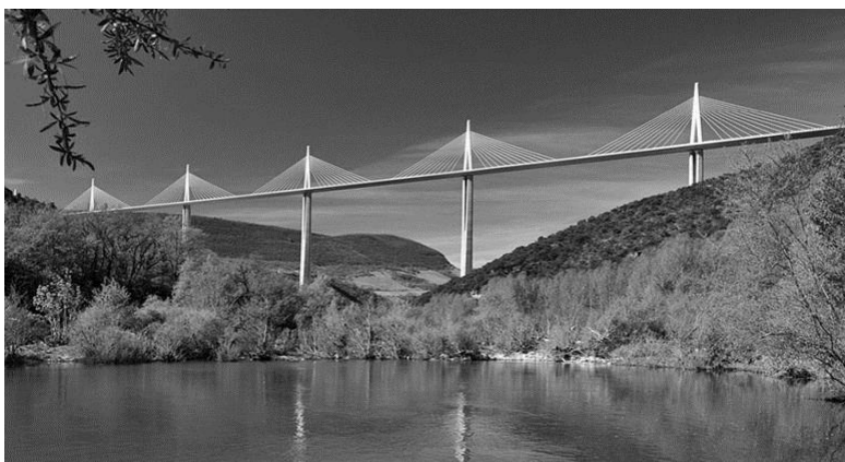
Fig. 4. Performance of a viaduct in Millau (France) with characteristic elements of a sketch and steel ropes upholding the bridge. Source: [21]
