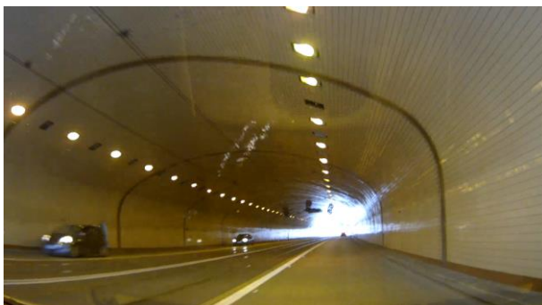
Fig. 10. Tunnel (unfavorable light)
