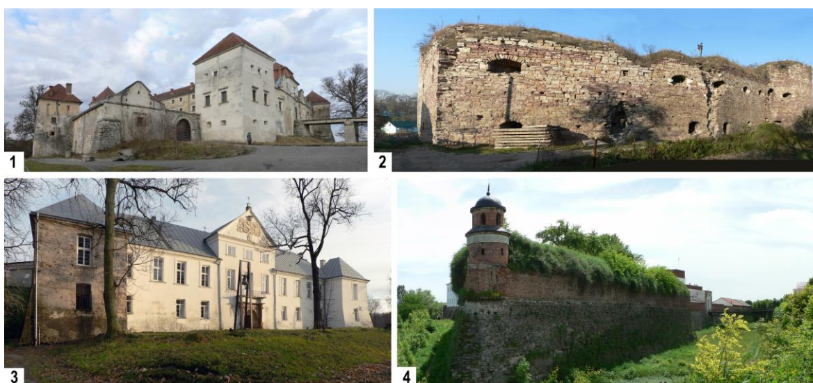
Fig. 4. Castles in 1) Svirzh (tower defensive system), 2) Buchach (bastei defensive system), 3) Yazlovets (2nd line) (early form of the bastion system), 4) Dubno (bastion system). Photo by O. Okonchenko
