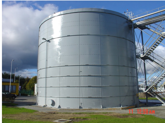
Fig. 18 Brine tank ( V = 2000 \text{ m}^3 )
