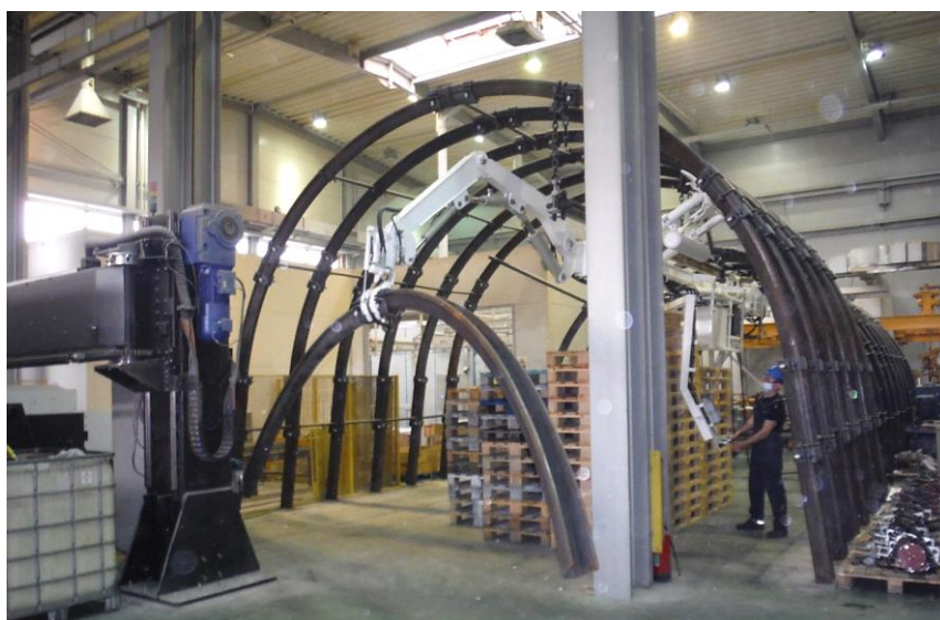
Fig. 8 Manoeuvring the support arch at the support frame installation site, with the use of (unfolded) stabilizing foot
