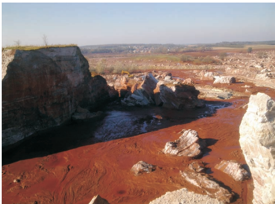
Photo. 2. The broken dam (inside view)
