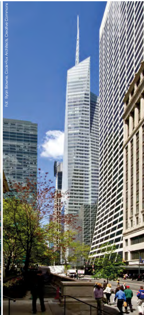
Fot. 3. Bank of America Tower
