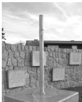
Fig. 7. New inox tube fixed at the base
