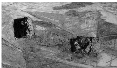
Fig. 4. Reinforcement of rotten parts with dowels and epoxy mass
