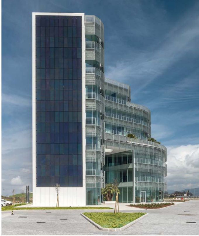
ill. 17: Forti holding headquarter south façade characterized by photovoltaic panels that provide 80% of electric power needs. (Credits: Photo by Irene Taddei, courtesy ATlproject).
