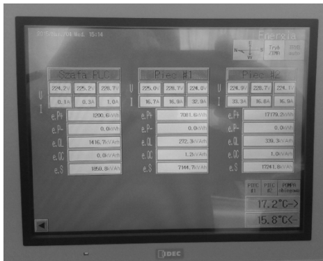
Fig. 3. Measurement of electric energy: a) N43 meters in electric furnaces, b) Operator panel with key data from N43 meters c) Operator panel with details of energy consumption for each phase
