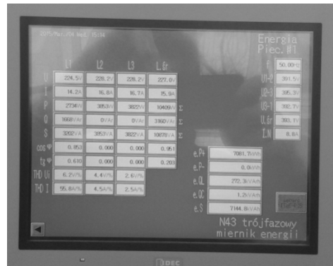
Fig. 3. Measurement of electric energy: a) N43 meters in electric furnaces, b) Operator panel with key data from N43 meters c) Operator panel with details of energy consumption for each phase
