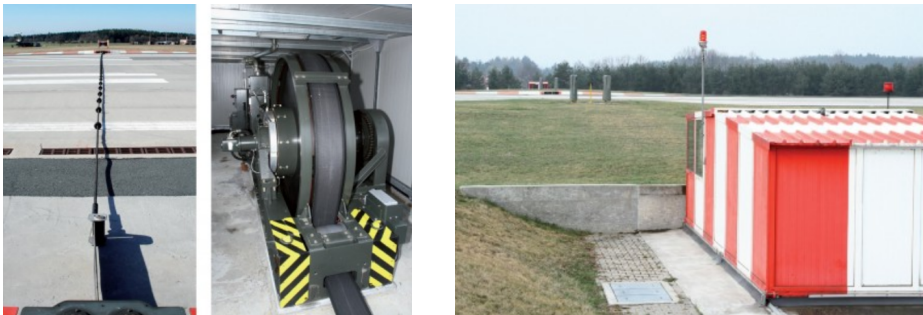
Fig. 12. Stationary devices of the BAK-12 arresting kit: view of the arresting cable, energy absorber and external ‘house’
