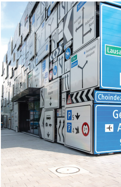
Exhibit 12. The building of the Swiss Museum of Transport, utilising old traffic signboards for the facade cladding. Design by Gigon & Guyer, Lucerne, 2009 ( https://image.architonic.com/imgArc/project-1/4/5204924/GigonGuyer-Verkehrshaus-der-Schweiz%2C-Luzern-04.jpg )
