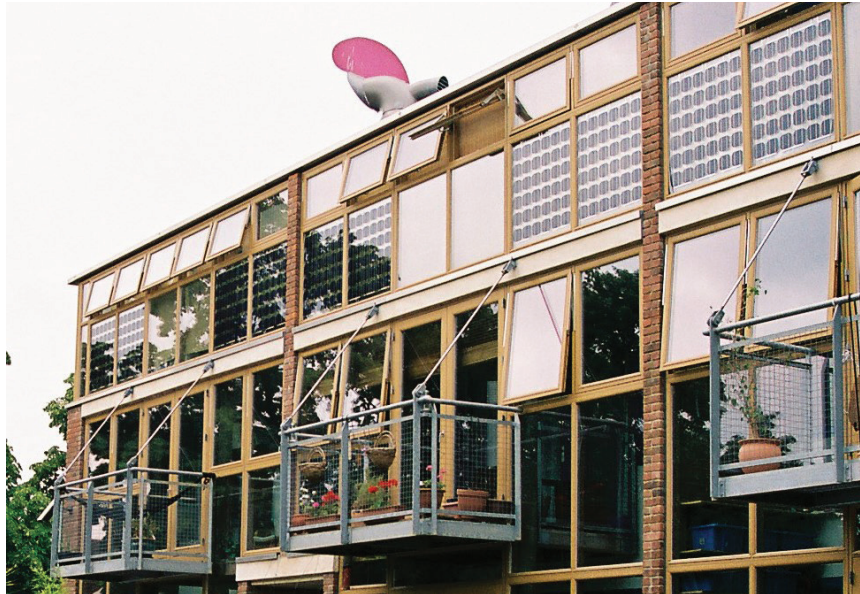
Exhibit 3. Photovoltaic cells printed on glass (the so-called Sky Gardens in BedZED village). Photo by A. Drapella-Hermansdorfer
