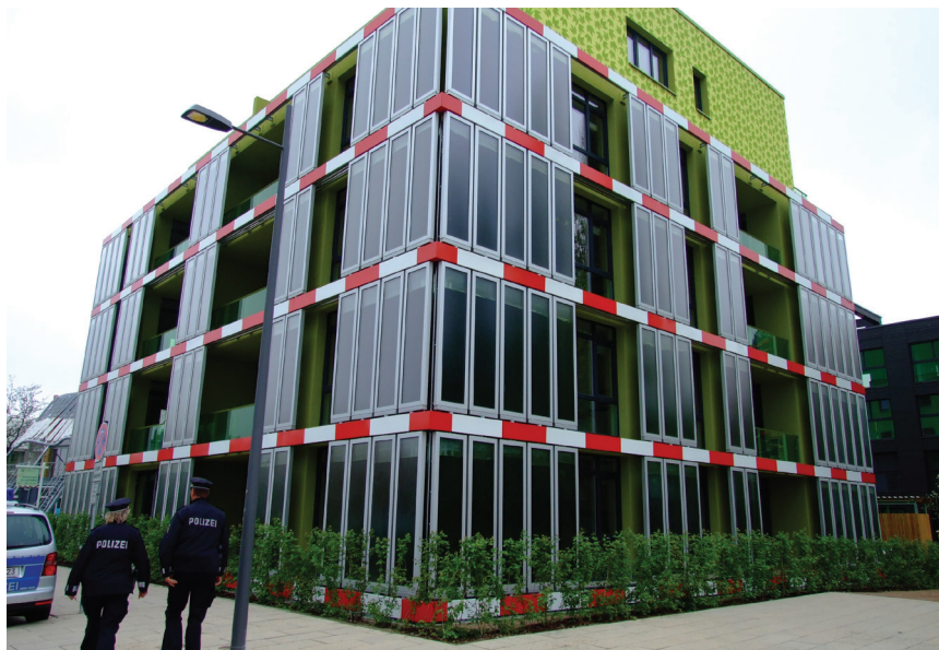
Exhibit 5. Building with bio-reactive facade, designed by Splitterwerk Architects and Arup, Hamburg, 2013. Photo by Author
