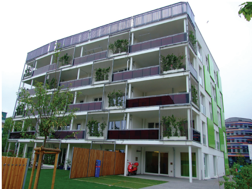
Exhibit 9. Smart is Green is an example of a three-layer facade building. Railing panels are filled with a phase change material (dark elements in the photo). Photo by Author
