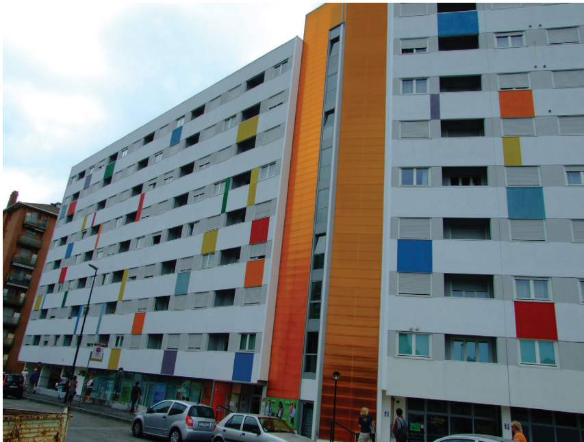
Exhibit 6. Casa Albergo – a building with façade partially painted with catalytic paints, designed by Studio Costa and Partners, Turin, 2011. Photo by Author
