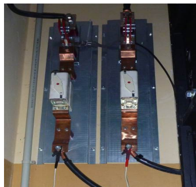
Fig. 3. Protection of energy storage device, a) High speed breaker BWS-1000[9]; b) Fuses and disconnectors at both poles of the battery [13]
