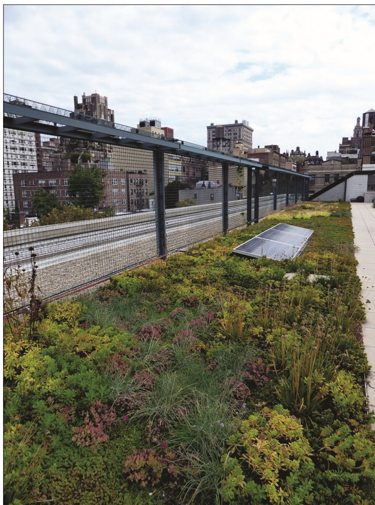
3. Zielony dach na Greenwich Village School w USA. Fot. Aloha Jon, 2016 r. 3. Green Roof on Greenwich Village School in USA. Photo by Aloha Jon, 2016
