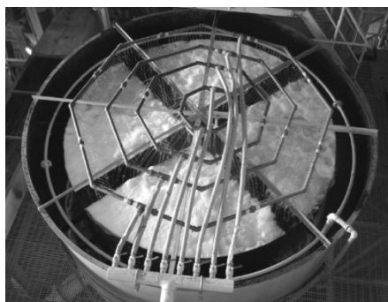
Fig. 3. Sarcheshmeh industrial plant flotation column
