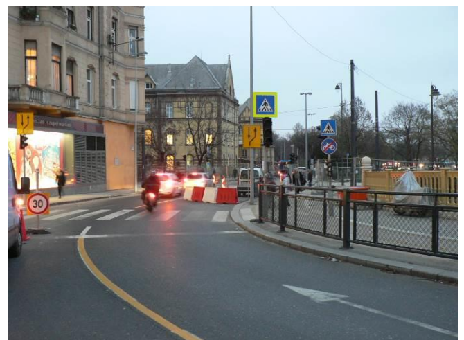
Fig. 7. Glued traffic markings used with old ones still visible
