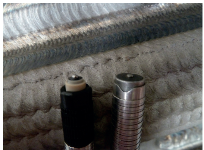
Fig. 12. Probes used to measure the thickness of the surfacing weld Source: own collections
