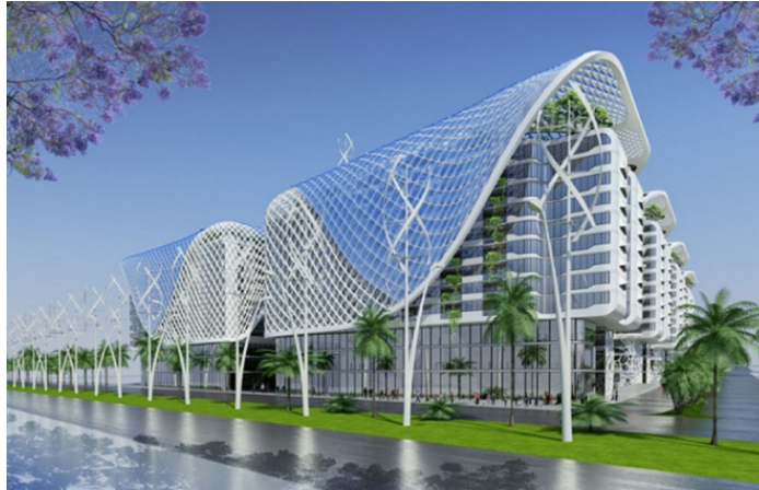
Fig. 6. “The Gate Residence” Project ( https://aasarchitecture.com ) (Egypt)
