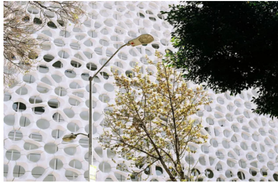
Fig. 2. Hospital building Torre de Especialidades (Mexico City) ( https://www.archilovers.com )
