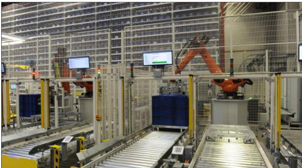
Fig. 4. Entrance part of automated small parts warehouse (AKL) with two robots
