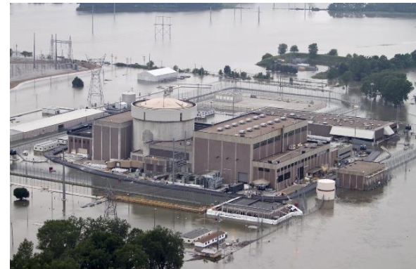
Figure 1. Fort Calhoun NPP site during the Missouri flood in 2011.
