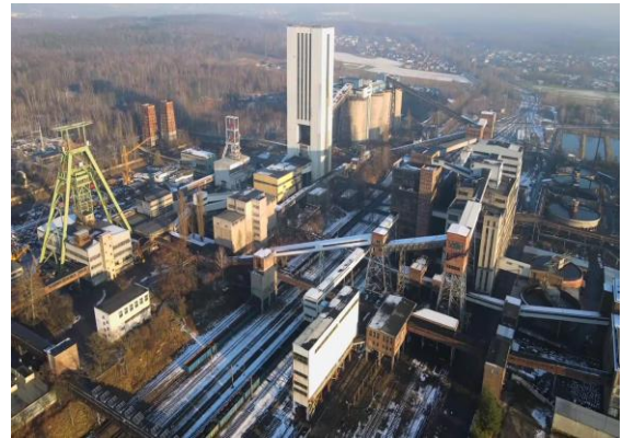
Fig. 1 Mine surface infrastructure facilities Y
