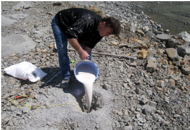
Fig. 1. Application of plaster paste to hole collar
