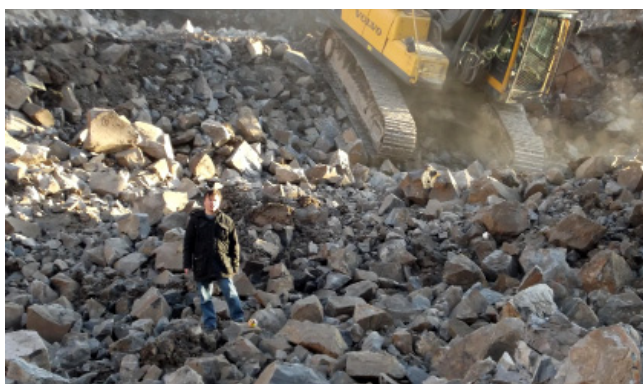
Fig. 5. Rock pile of blast round with plaster stemming at Asagi Caglayan basalt quarry
