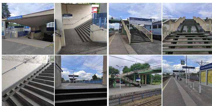
Fig. 1. The main railway station in Bielsko-Biała –access to the platform, the shed, and the footbridge (the authors’ photography)
