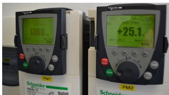
Fig. 3 Setting the entry speed and torque on frequency inverters Altivar
