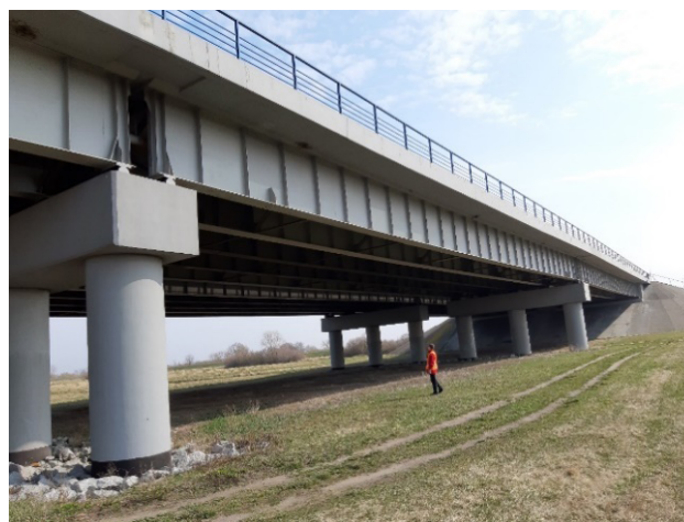
Figure 1: View of selected spans of the bridge structure.
