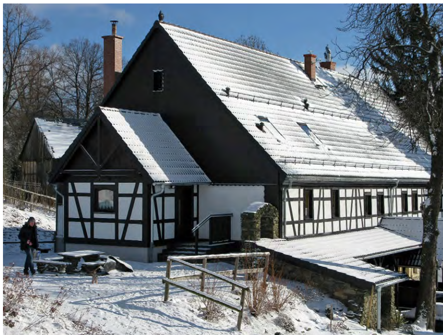
Fig. 2. Newly renovated, maintaining the original architecture, building in Dziwiszów (now agrotouristic venture) (photo by Ewa Malec-Wysocka)
