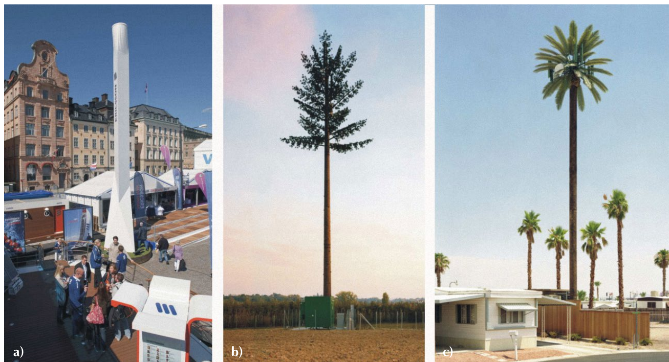
Fig. 4 a–c. The telephone masts of cellular telephony; and) in city, b–c) in open terrain
