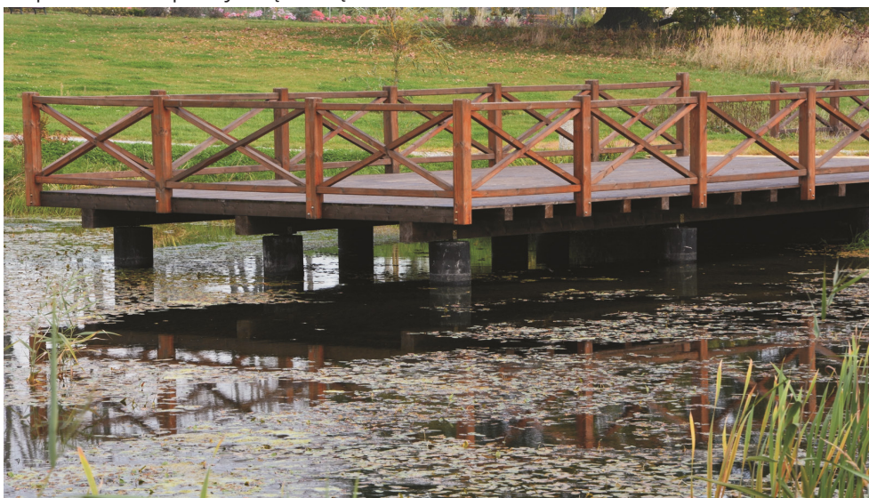
Fot. 5. Platforma widokowa posadowiona na palach. Pic. 5. View platform founded on pickets.
