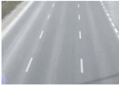
Fig. 1. Test road section with “even” surface (asphalt)
