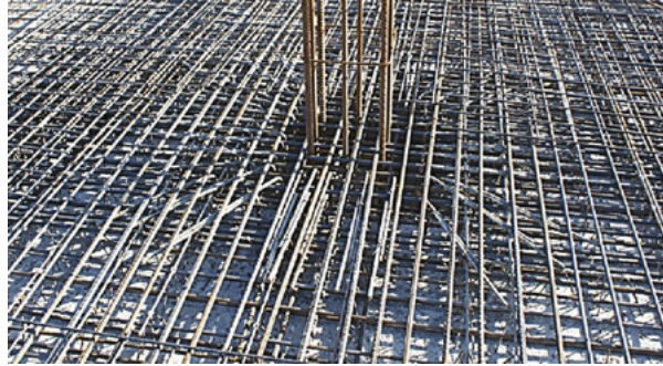
Fig. 17. Detail of the reinforcement in the vicinity of support
