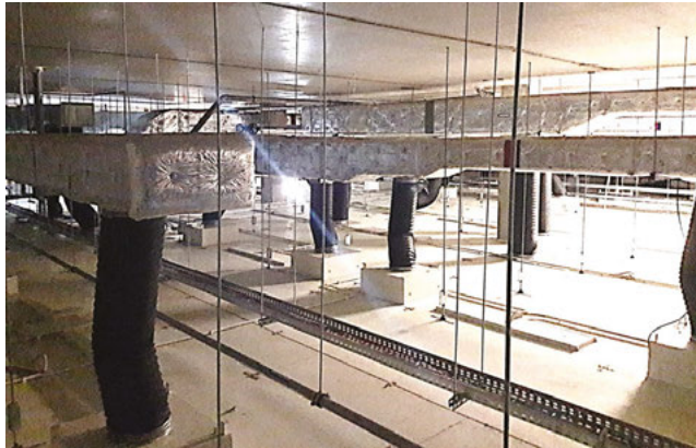
Fig. 12. View of the space between the floor slab and a suspended ceiling with technical equipment
