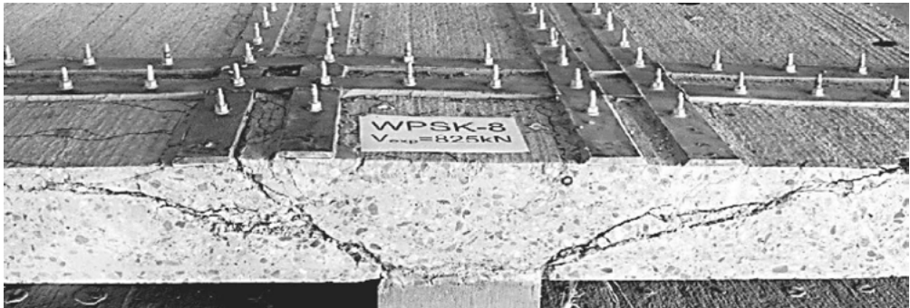
Fig. 10. View of the saw-cut of the specimen after failure [17]
