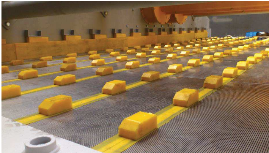
Fig. 9. Installation of deck in the PWP1-2.4x5.25 screen
