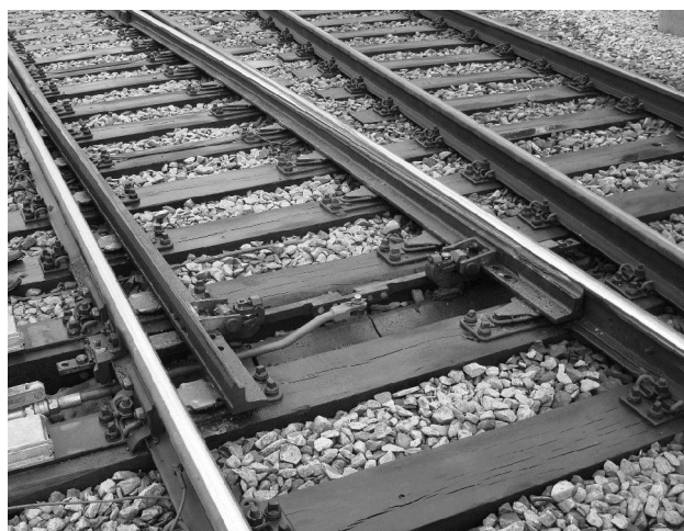
Fig. 2. Ordinary turnout switch panel [photo. M. Czarnecki]
