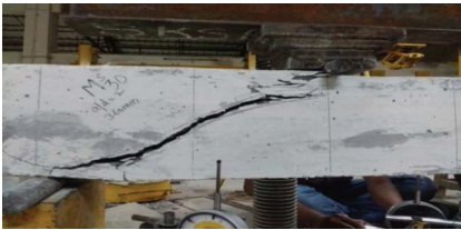
Figure 10 Failure pattern of SCC30
