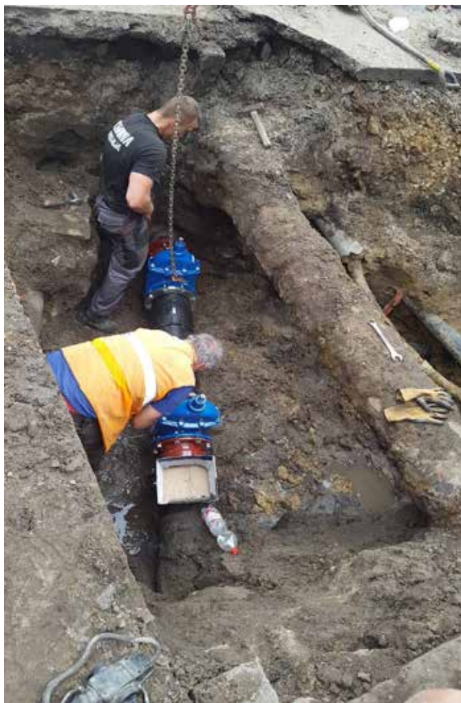
Fot. 7. The successive stage of gate tee replacement
