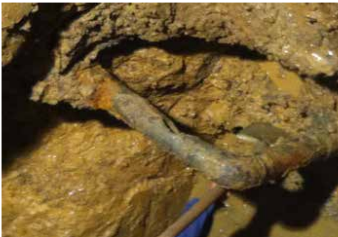
Fot. 5. Damage of steel connection during performance of jacking
