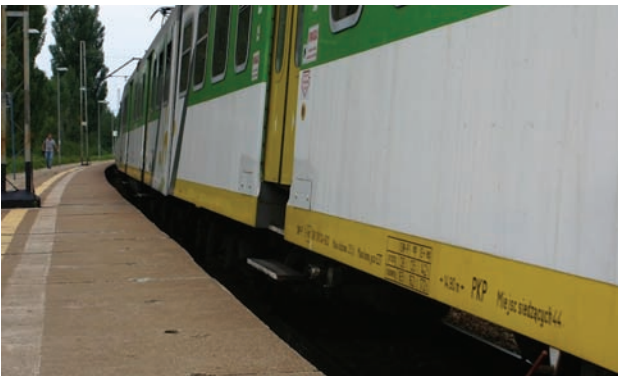
Fig. 3. The no longer existing platform at one of the stations in Mazovia with the edge of the platform clearly away from the train [photo by G. Stencel]
